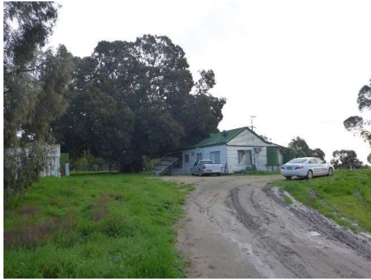
Plate 9. View north towards existing residential house on Lot 3/ DP 562598.
