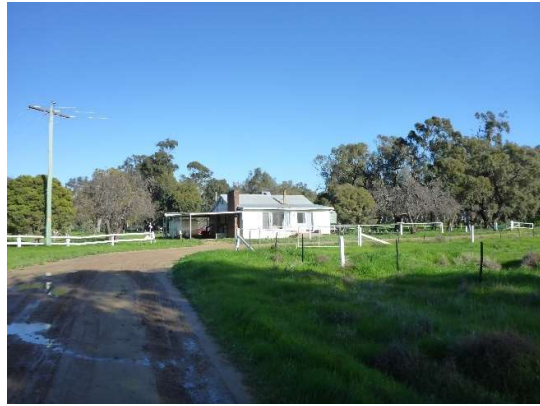
Plate 10. View south towards existing residential house on Lot 1/ DP 1121183.
