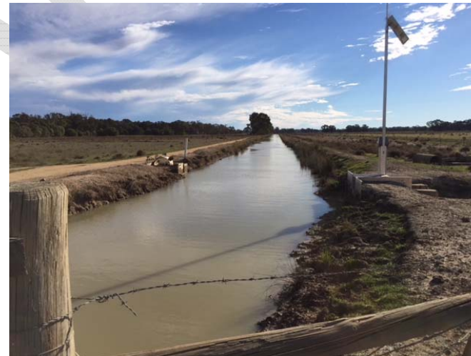
Figure 2-4 Irrigation Channel (Source: GHD)
