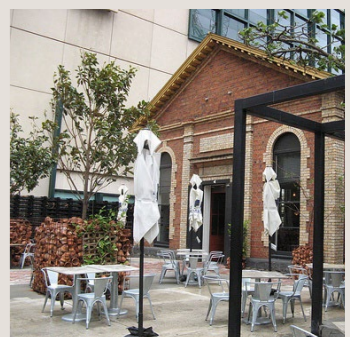
Adaptive reuse of existing building - Hebrew School by Heritage Victoria
