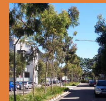
Victoria Square Water Sensitive Urban Design (WSUD) directs stormwater to central median
