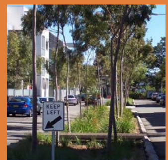
Victoria Square Water Sensitive Urban Design (WSUD) directs stormwater to central median
