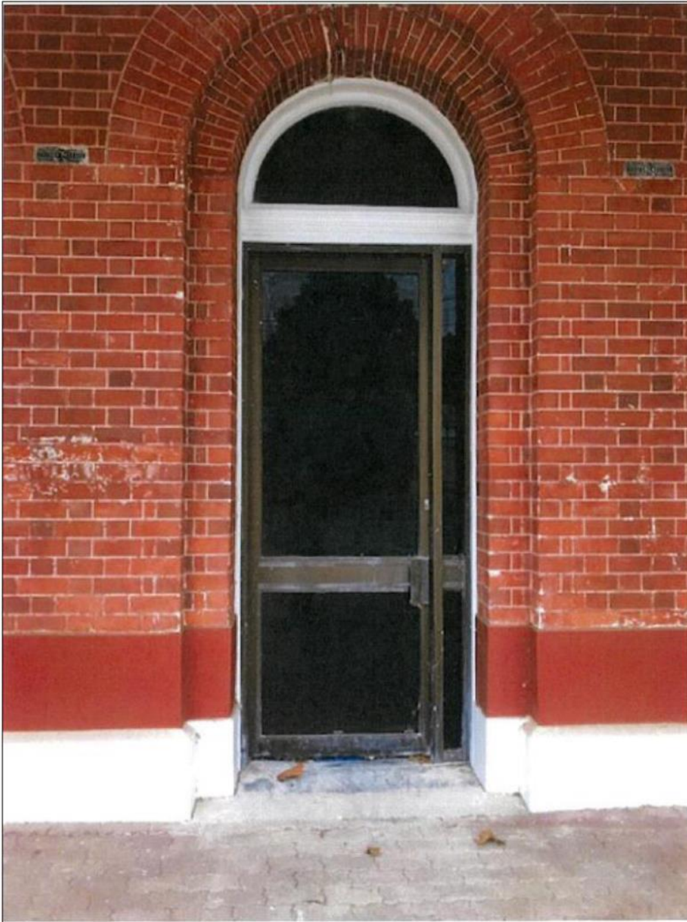
Figure 6 Front door at 138 End Street
