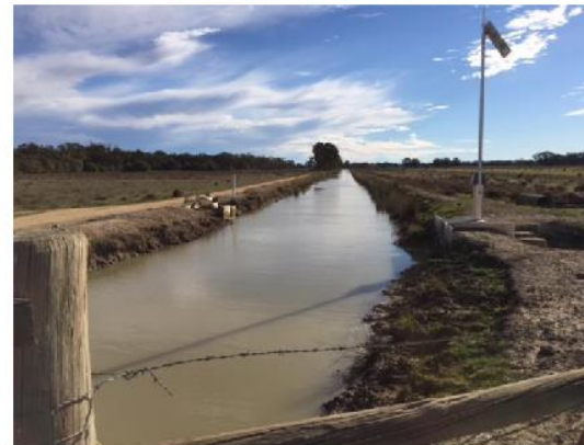
Figure 2-4 Irrigation Channel (Source: GHD)
