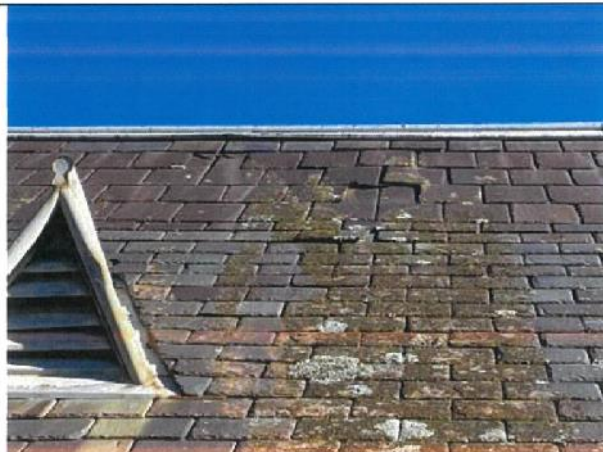
Photograph 10 Missing slate and loss of fixing
