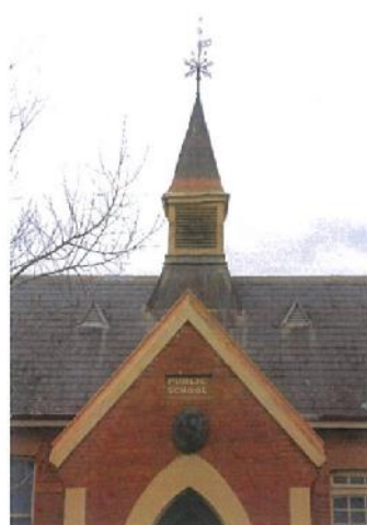
Photo 14: view of former entry, parapet & spire
