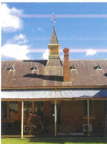
Photo 13: view of verandah, roof vents & spire
