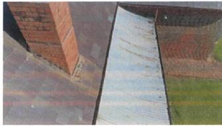
Photo 9: view of roof conditions
