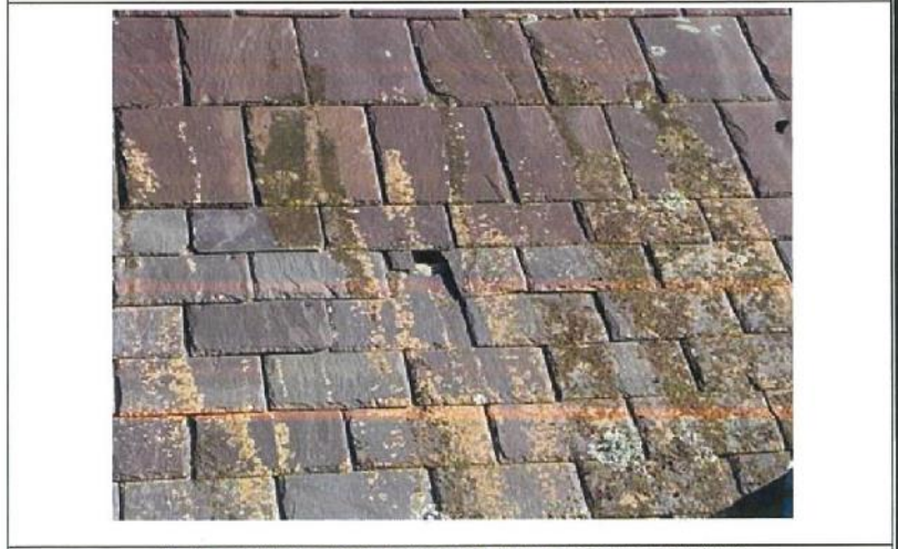
Photograph 2 Broken slate typical and smaller slate tile to southern half of roof
