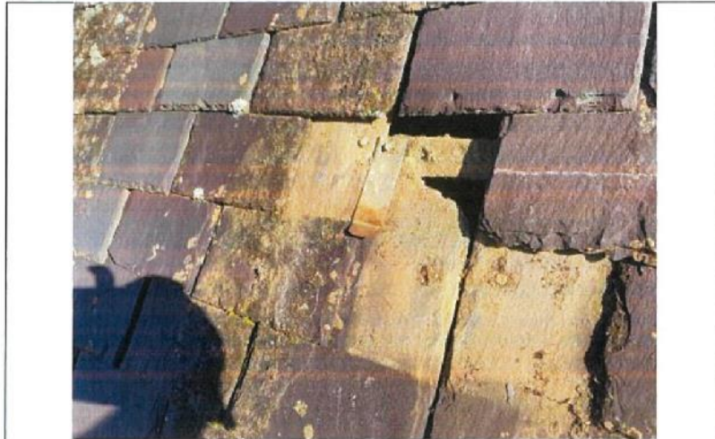
Photograph 15 Popped and corroded galvanised nails and clips
