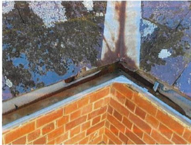
Photograph 20 Slate not finished to eave gutter correctly and back of eave gutter cut out
