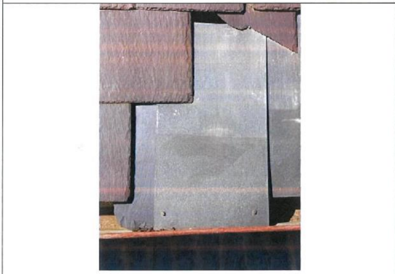
Photograph 24 Painted flashing that has let go
