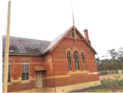
Photo 2: view of front - east side of building
