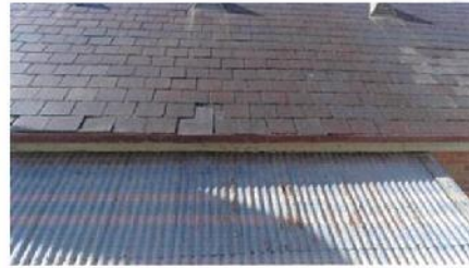
Photo 10: view of roof conditions
