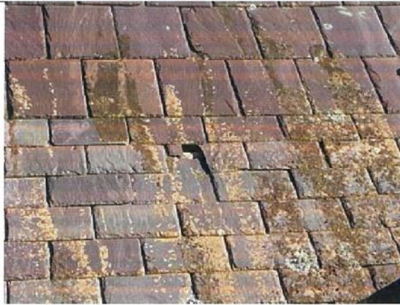
Photograph 13 Broken Slate
