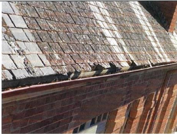
Photograph 9 Loose slate at fascia / eave gutter
