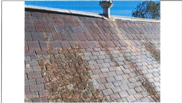
Photograph 5 Loose ridge roll capping
