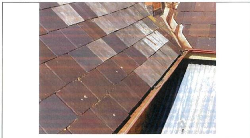
Photograph 25 Painted flashings used for slate replacement
