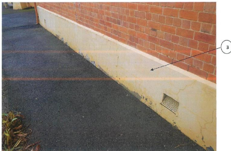
Photo 6: Peppin Heritage Centre (former Public School) – view of rendered base plinth
