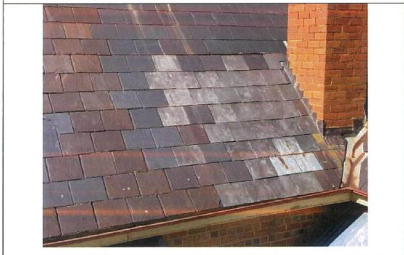
Photograph 22 Painted flashings used for slate replacement
