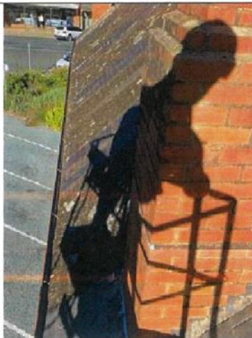
Photograph 4 Chimney flashings and moss growth
