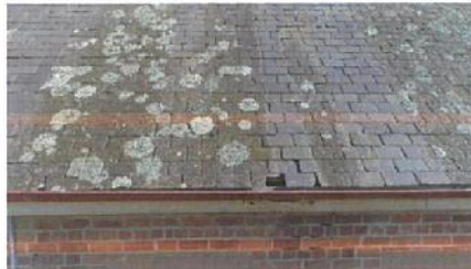
Photo 6: view of roof conditions
