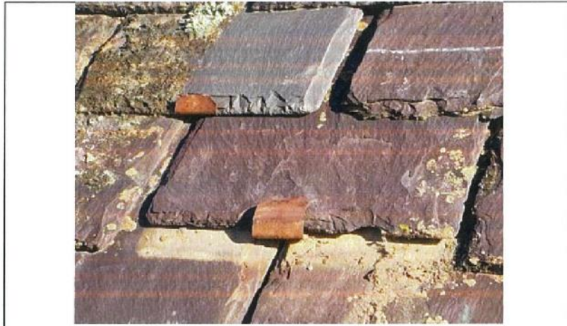
Photograph 11 Corroded clips where repairs have been affected
