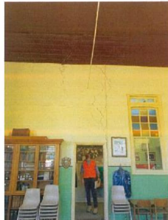
Photo 20: view of classroom wall - cracking
