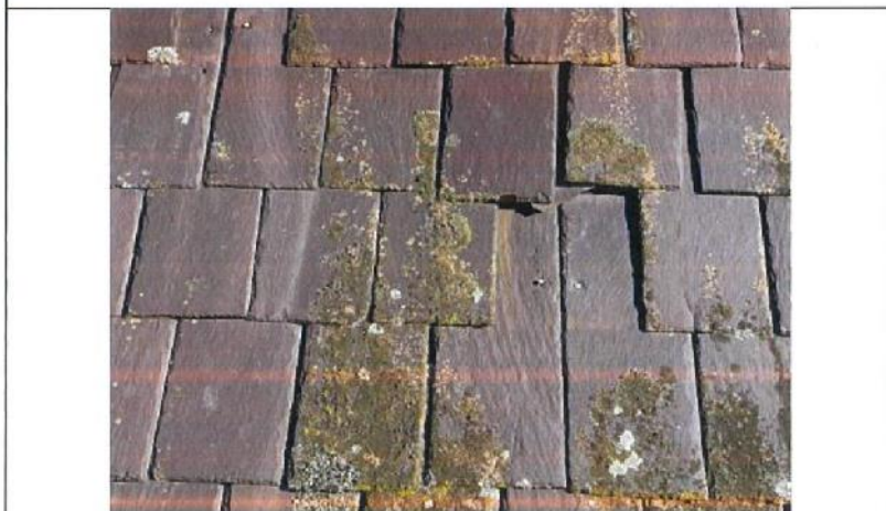
Photograph 12 Broken / missing slate
