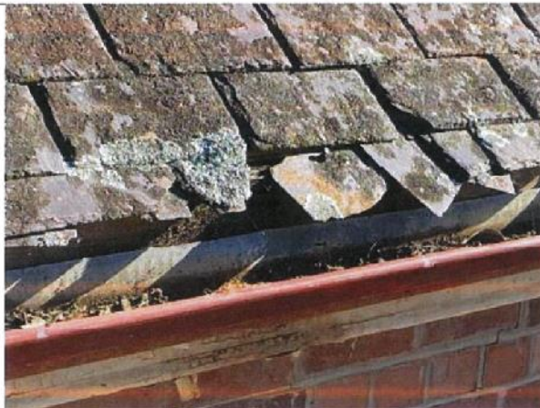
Photograph 8 Loose slate at fascia / eave gutter
