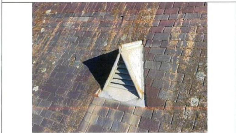
Photograph 6 Dormer vents in okay condition
