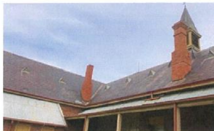
Photo 8: view of rear verandah and roof
