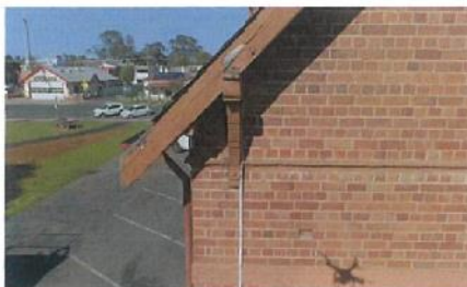
Photo 7: view of front of building
