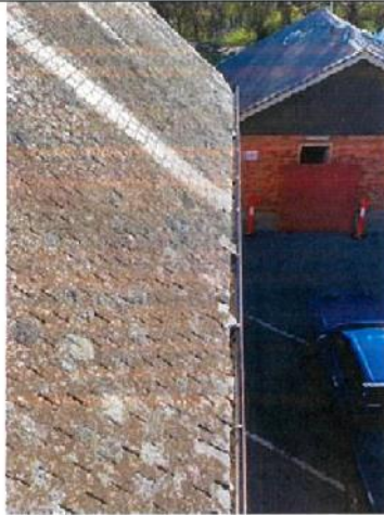
Photograph 3 Slates that have let go and slipped into eave gutter
