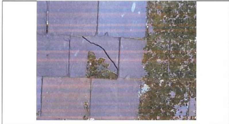
Photograph 17 Cracked slate
