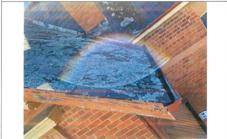
Photograph 16 Rotten barge and moss build up
