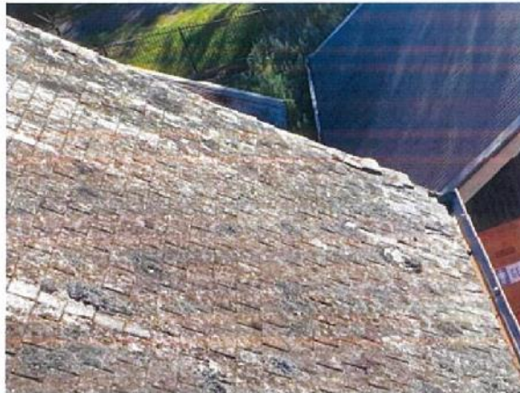
Photograph 7 Loose slate at barges
