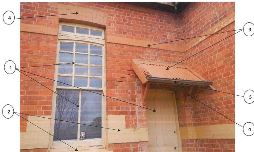
Photo 5: Peppin Heritage Centre (former Public School) – view of window, door and canopy
