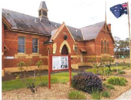
Photo 1: view of front of building
