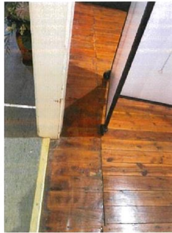
Photo 24: view of gallery flooring
