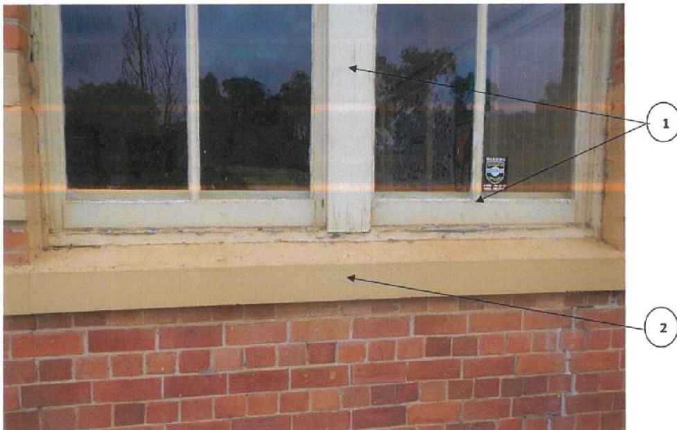
Photo 4: Peppin Heritage Centre (former Public School) – view of windows & rendered sills
