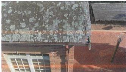
Photo 5: view of roof conditions
