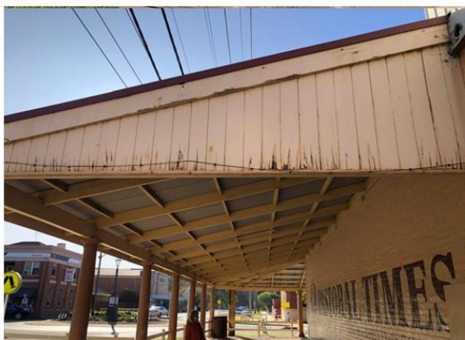
Figure 15 – Boards require Sanding & Repainting
