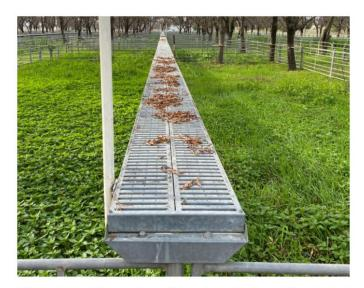
This can be rectified by dismantling and reusing the existing planks. The cross supports on the top of the posts will need to be remade to cater for the addition of another plank and to hold the stanchions. Hand and knee rail running horizontally can then be installed.
