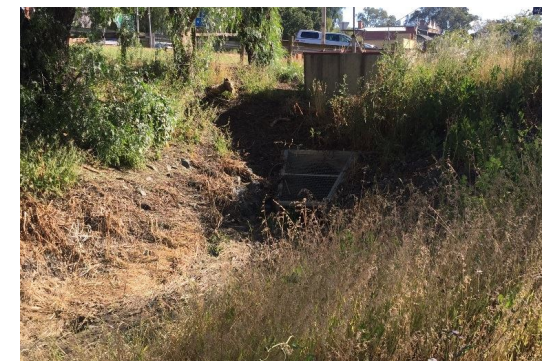
Pipe through South Deniliquin Levee
