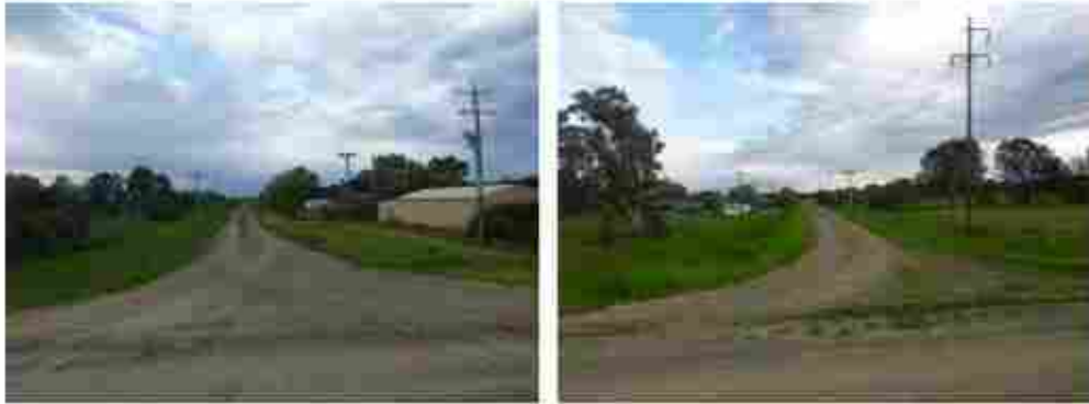
Plate 4-5 Views of Section 8: from the northern end looking south-east (left), and from the southern end looking north-west (right).
