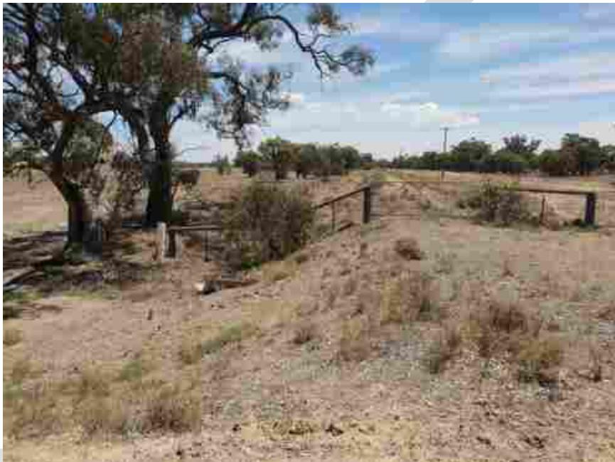
Figure 19: Levee north of Smart Street to be raised 200mm
