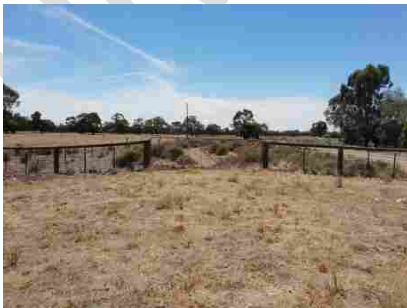
Figure 20: Levee north of Cobb Highway to be raised 200mm
