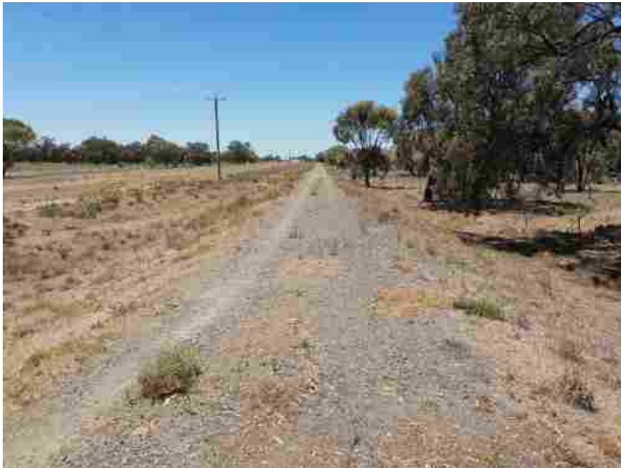
Figure 16: Looking South-East along Flanagans Channel Levee from Smart Street
