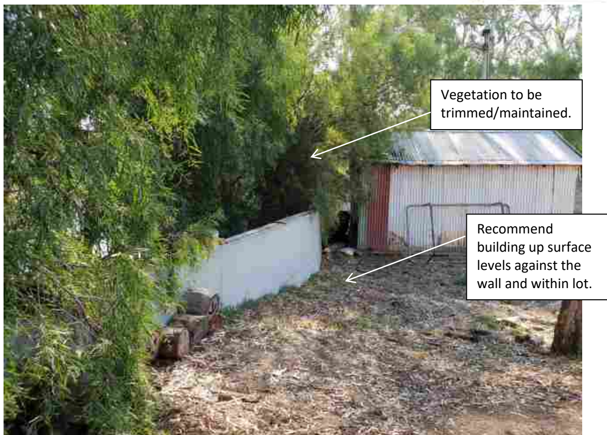
Figure 34: Photo looking at CH 570 where concrete wall is highest above surface level.
