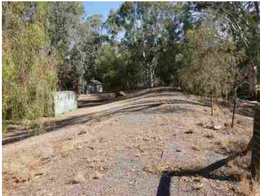
Figure 31: Looking South CH500 along Hyde St bank
