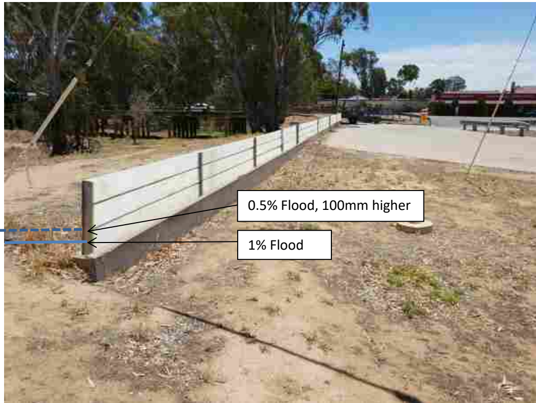
Figure 29: Realistic impression of sleeper retaining wall on existing wall.
