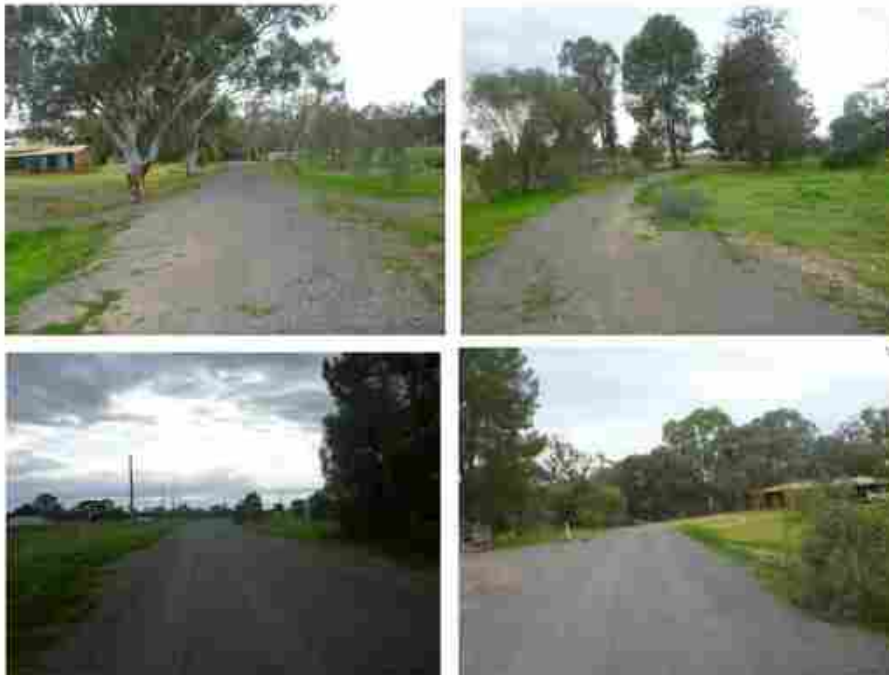
Plate 4-1 General views of Sections 2 and 3: the central part of Section 2 (top left), the northern end of Section 2 (top right), the eastern end of Section 3 (bottom left), and the western end of Section 3 (bottom right).
