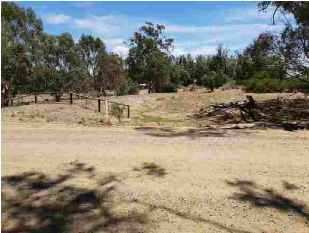
Figure 24: Levee through No: 156-168 April Street onto Smart Street.
