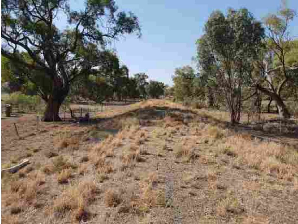
Figure 12: Looking North CH 480 Section 2
