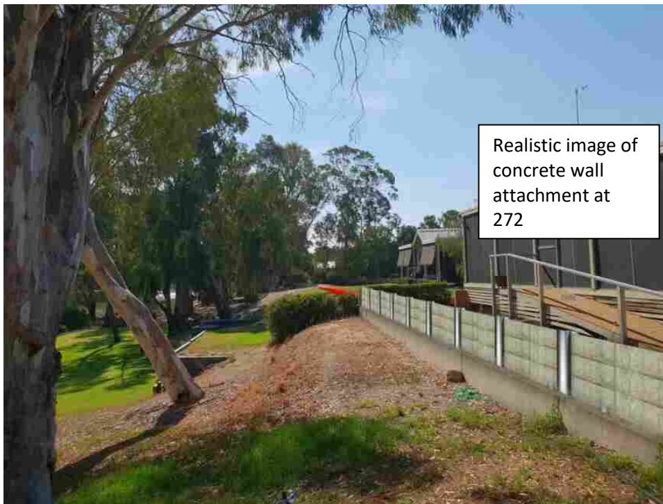
Figure 38: Image of wall at 272 River Street
