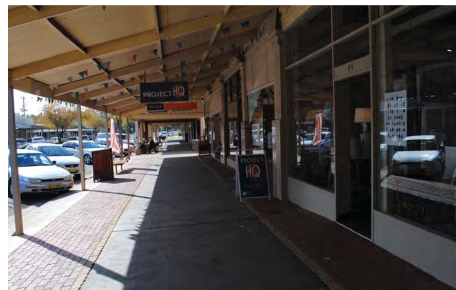
Existing foot path condition
