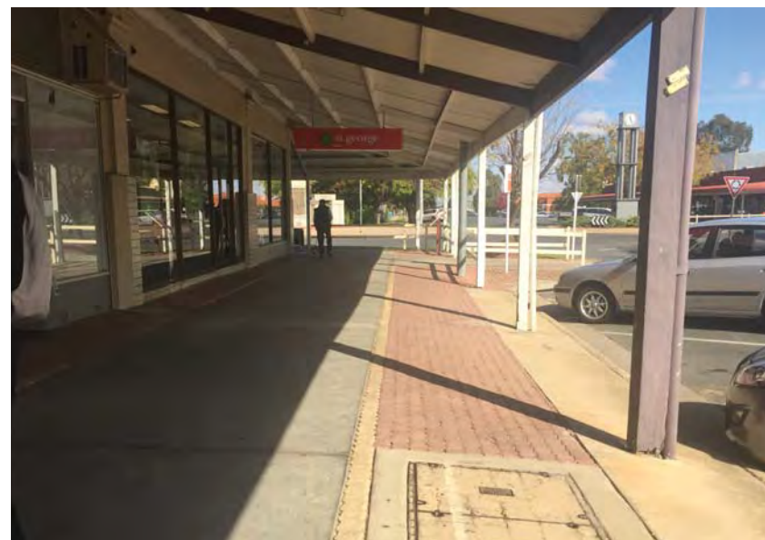
Existing foot path condition
