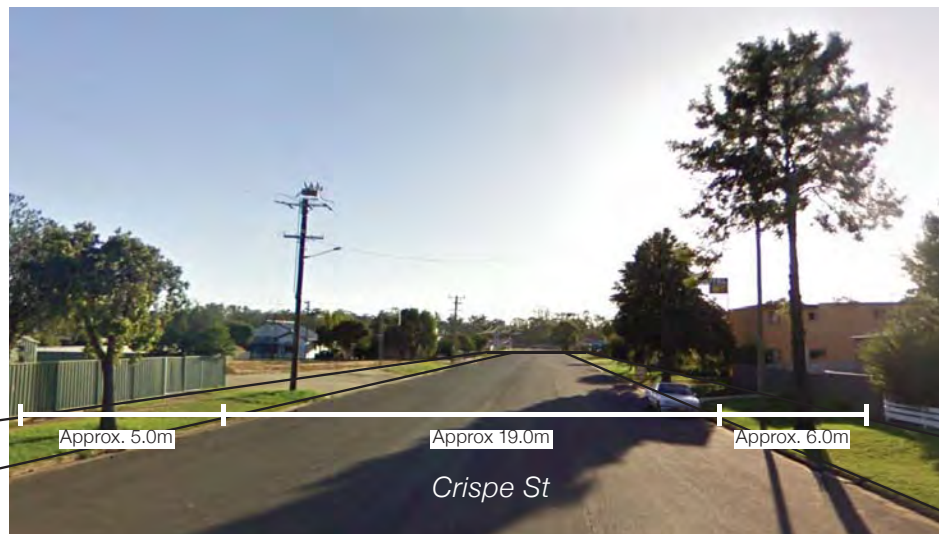
Existing Road Reserve (Google Street View)
