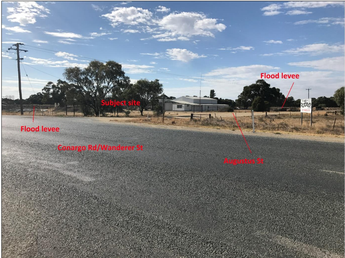
Photo 3 Subject site from Conargo Road/Wanderer Street looking north east
