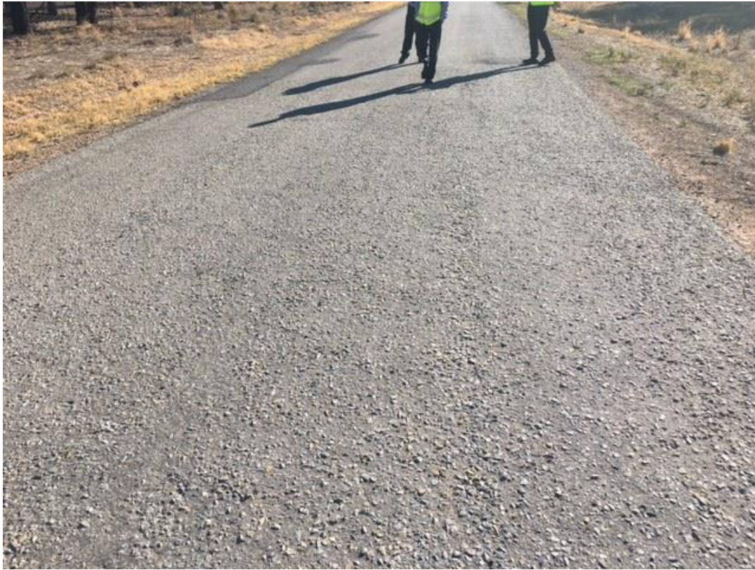
Recently completed OTTA seal Road
