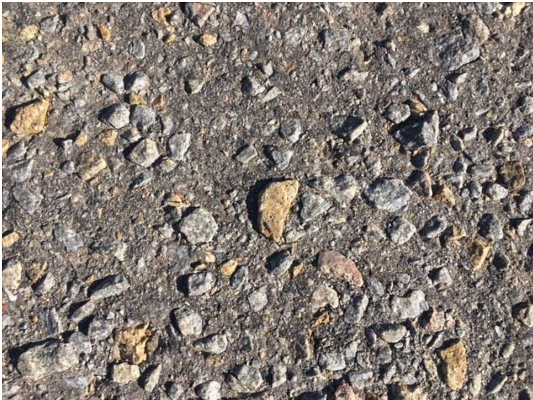
Rough stone on surface of OTTA sealed road
