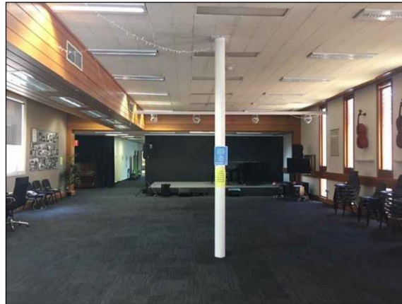
EXISTING CONCERT HALL TO BE UPGRADED
