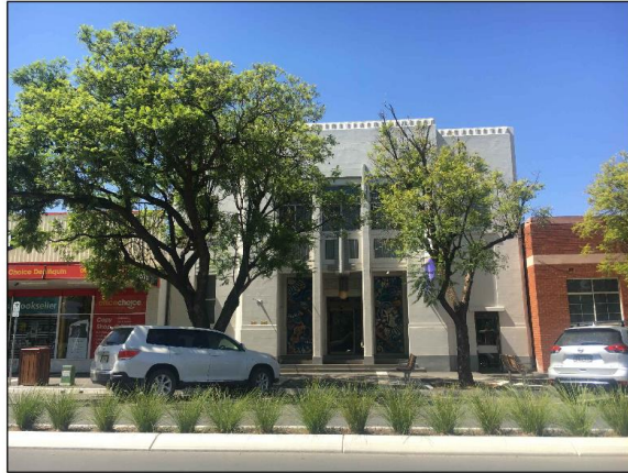
FRONT VIEW FROM CREEY ST
