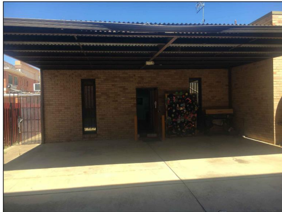
VIEW FROM REAR CAR PARK
