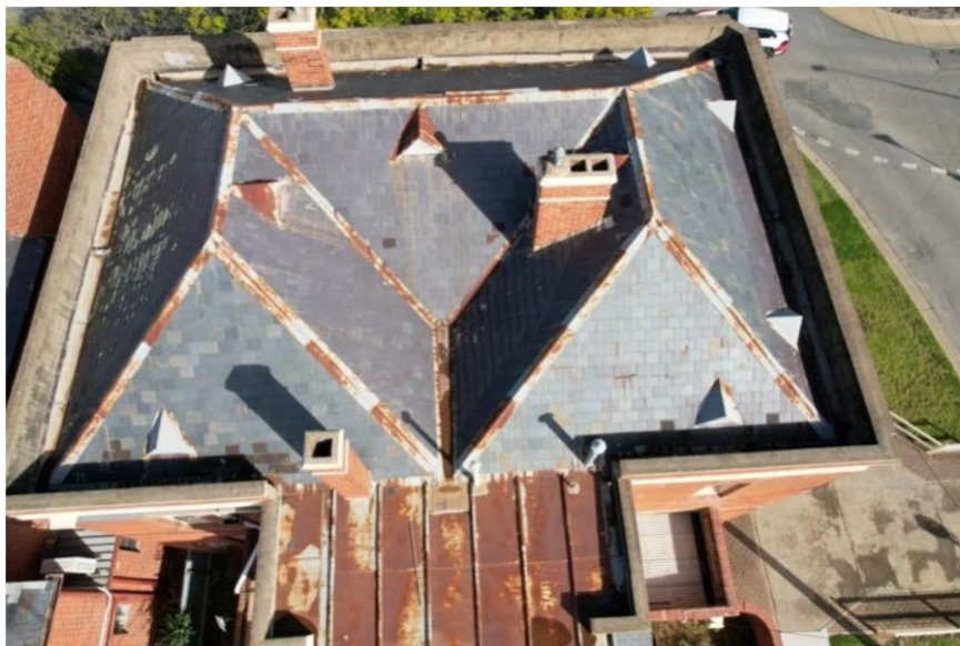
Figure 6: View of the slate clad hip and valley roof taken via drone.
