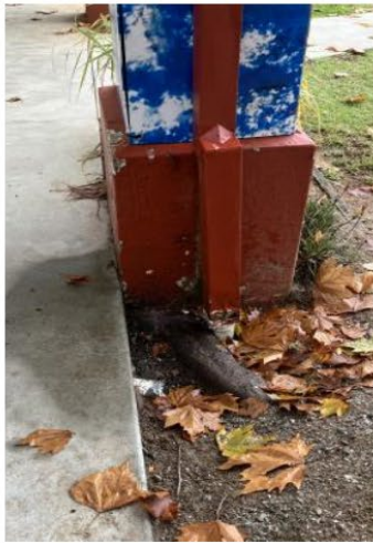
Tree root undermining building columns
