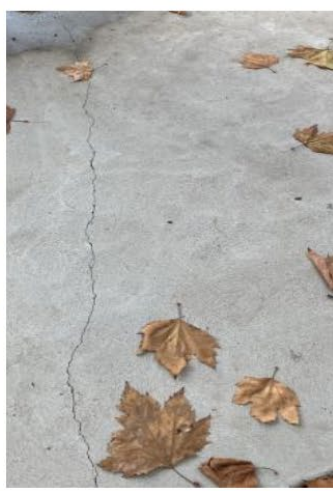
Surface cracking in pavement potential displacement
